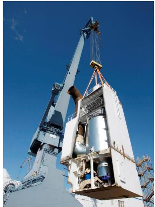
Installation of a closed loop scrubber system
