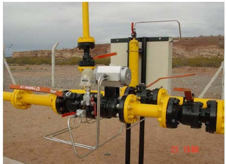
Honeywell wireless transmitters monitor pressure transmitter WG514 in fuel gas pipeline.
