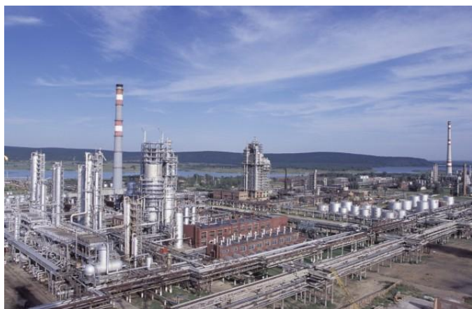
Angarsk Refinery, Irkutsk Region (Eastern Siberia).
