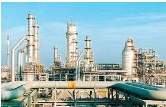
ONGC's Hazira Gas Plant in India
