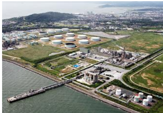
Taiyo's Yamaguchi Operations, located in Ube City, Yamaguchi Prefecture, Japan.
