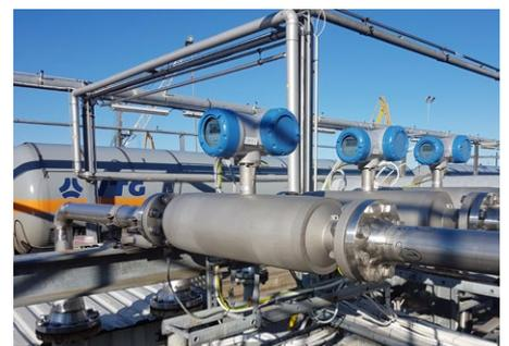
Figure 3: Coriolis flowmeter technology provides accurate and reliable mass flow readings.
