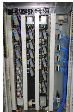
Experion LX Control Rack at LGLS
