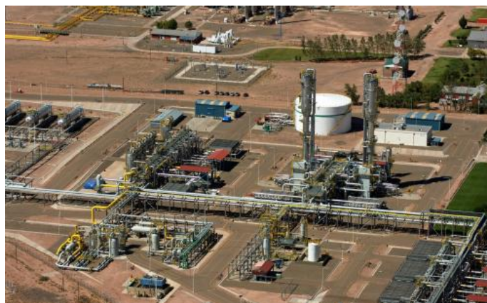
Aerial view of natural gas separation plant at Loma La Lata, Province Neuquén, Argentina
