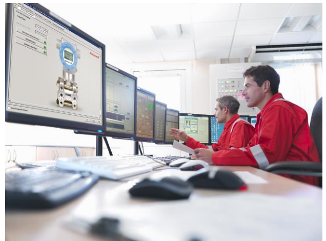
Combining the Experion control system with SmartLine transmitters helps plants improve their efficiency.
