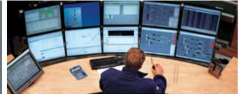
Fault Tolerant Ethernet (FTE) is the control network of PlantCruise. FTE is dedicated to providing not only fault tolerance, but also the performance and security required for industrial control applications.
