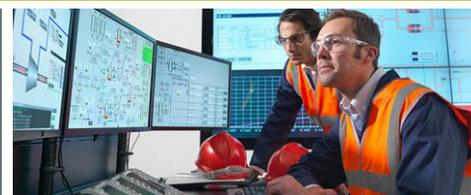
DynAMo® notification is separate from the alarm system enabling operators to benefit from information during normal operating conditions without being overwhelmed by it during process upsets.
