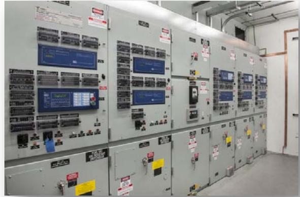
Figure 6, Typical Switchgear with IEDs in a Substation
