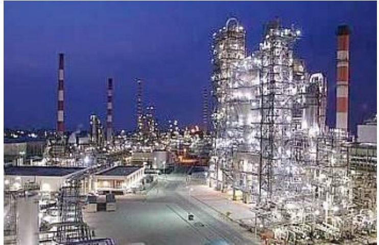
Fig. 5. Refining and petrochemical facilities must be particularly diligent about operations monitoring for productivity, reliability and safety reasons.
