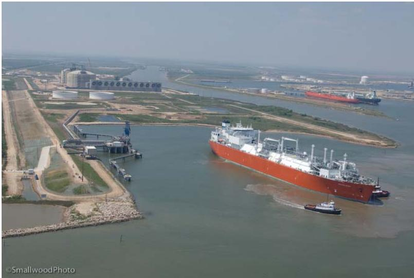
Phase one of the terminal construction, which began in January 2005, included two 160,000 cubic meter LNG storage tanks, vaporization facilities, as well as the piled unloading dock for handling LNG vessels. The first phase of the project allows the facility to have a send-out capacity of 1.75 Bcf/d peaking.
